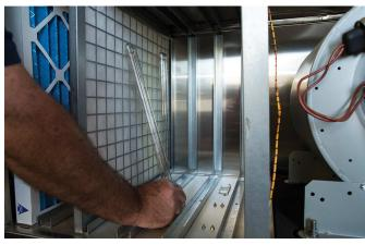
4. Install by holding on the base only. Lean bulb over in the direction of the safety latch on the socket, insert the bulb and then straighten bulb as it inserts into the bulb socket.
